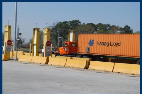
**Passive Radiation Detection Equipment**
